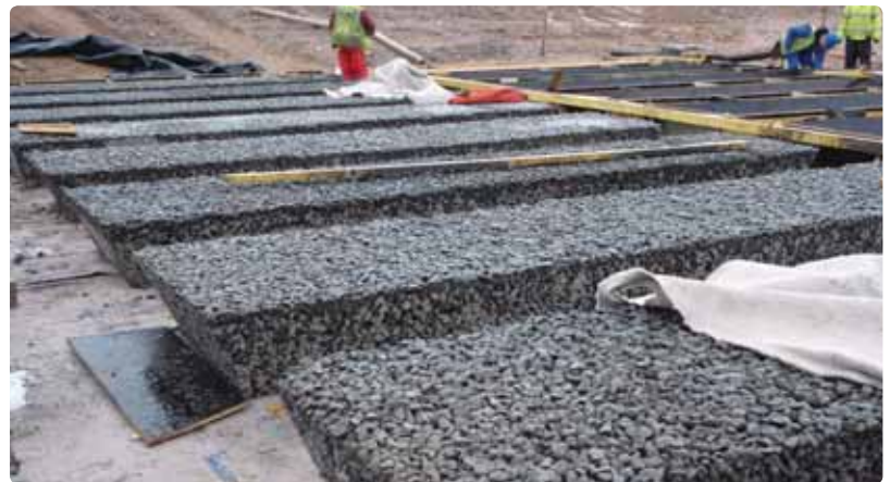
Figure 4 below: In-situ topping to the concrete elements.
