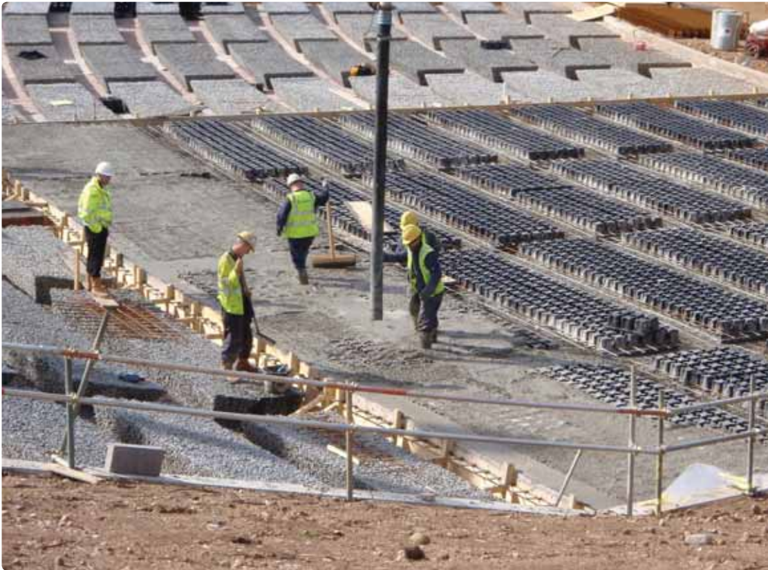
Figures 2 and 3: No-fines concrete elements seen at distance.
