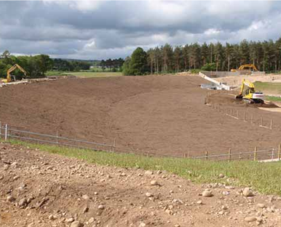
Figure 1 above: Spillway and stilling basin.
